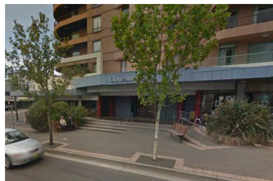
Borrodale Rd – public domain upgrades
